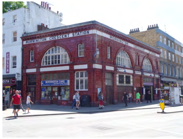
Typical Early Station
